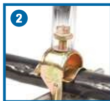
2 Using a power tool fitted with a 1/8" (16mm) socket, tighten lock nut...
