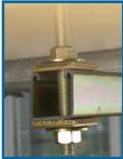
Standard method using nuts and washers.
