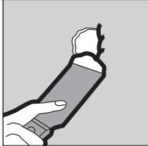
Trim any loose material and wipe area clean. Apply generous amounts of joint compound around edges and coat the perimeter of hole.
