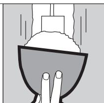
Apply compound over tape with knife. Let harden and apply second coat of compound if necessary. Sand and prime when dry.
