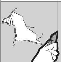
Cut a section of new wallboard larger than the hole. Position the wallboard over the hole, trace the wallboard's shape onto the wall. Use a jab saw or utility knife to cut out the outlined section. Remove old fasteners.
