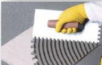
Apply the mortar to the back of the ceramic tile with the smooth side of the trowel forming strands parallel to the notched part of the band.
