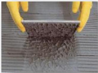
During application, randomly remove some tiles and check that the mortar strands are being broken.
