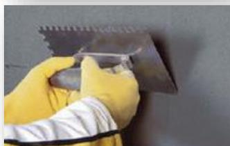
Apply the mortar (thickness 3mm to 4mm) with the smooth side of the trowel. Roll out one small area at the time to prevent the mortar from drying out. See manufacturers information.
