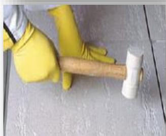
Apply the tile piece slightly out of position, crossing the strings of the back of the tile and the subfloor. Drag the tile piece to its final position by finger-pressing and tapping with a rubber hammer to knead the mortar strands.
