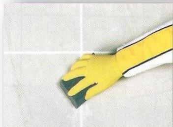
Finish with clean, slightly wet sponge no later than 30 min after grouting.
