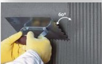
Pass the toothed side of the trowel (8mm x 8mm x 8mm) at an angle of 60 ° to the base, forming parallel cords and grooves.
