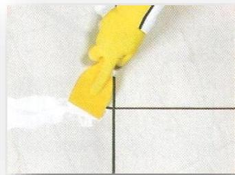
Spread the grout on the grout lines using a rubber spatula.
