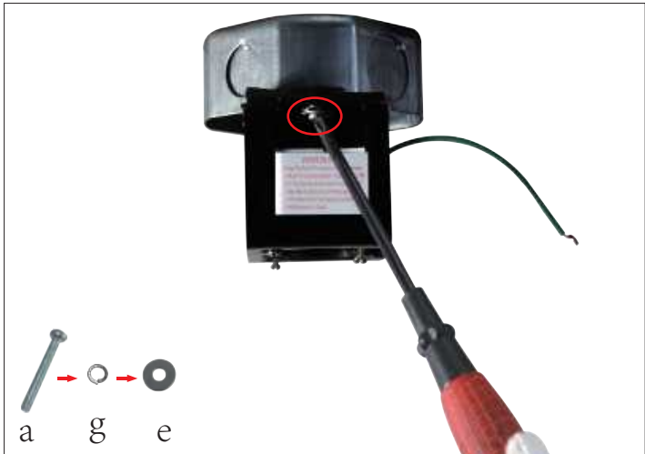
Step 1 For concrete ceiling, install the mounting plate to octagon box with two machine screws.
