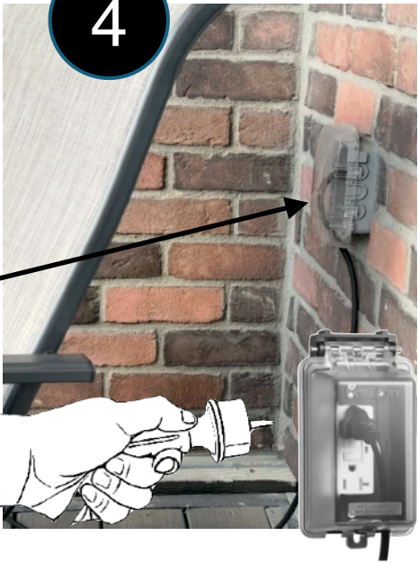
Plug in the inverter cord to a 120V weatherproof outlet
