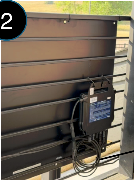
Secure Micro-Inverter to balcony with supplied cable zip ties
