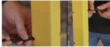
**6.** Using the hex key stored on the collar assembly, tighten both set screws on the split boom connector securely.
