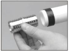
Slip a copper crimp ring onto the tube, and insert tube up to the fitting shoulder.
