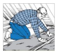
When using insulation batts, place them one after the other until you reach the center. Simply cut the insulation to fit. Install insulation the same way on the opposite side of the attic, working from eaves toward center.
