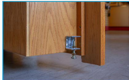
Outswing, support bolt bracket
