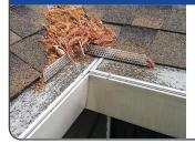
Roof valleys can cause excessive rain water and debris build up creating challenges for all gutter guards. Rainwater diverters help hold debris back and away from the gutter guard.
