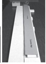
NOTE: The heating blankets <u>must not</u> touch each other. Place scrap pieces of trim between blankets if necessary.
