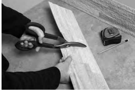
Cutting a straight cut with a snip
