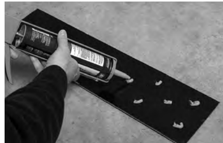
Method 2 - Using high-quality polyurethane construction adhesive
