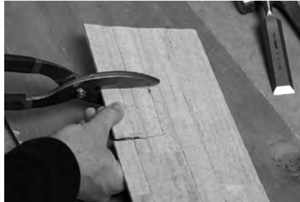
Starting a notch using a snip
