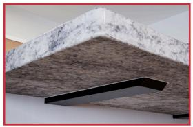
5. With your countertop now resting upon the brackets, we recommend applying a bead of clear silicone adhesive around the brackets.
