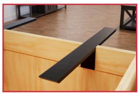
2. Once your cabinet is notched, place your bracket within the notch, so as the bracket's vertical support is on the inside of the cabinet.
