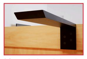
3. Once your brackets are in place and level, drill pilot holes through the holes on the bracket. Once pilot holes are made, drill the screws through the pilot holes, fastening the bracket to the inside of the cabinet.
