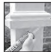
7. Caulk gaps between shaft and cap and base as desired.
