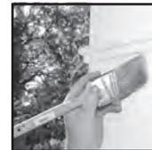
8. Paint with a high quality oil or acrylic latex paint. Remove all dust and dirt by thoroughly wiping column with cleaner compatible with your chosen paint (mineral spirits for oil paint, Simple Green® or isopropyl alcohol for acrylic latex paint.) Allow to dry completely before painting.
