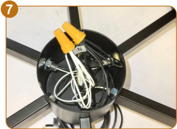
Use the wire connectors in the accessory kit to secure it.
