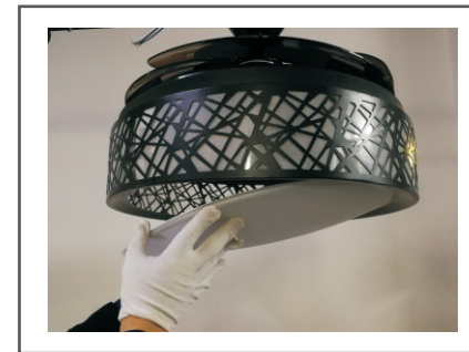
Step 6. Place the acrylic panel gently into the lampshade holding slot.
