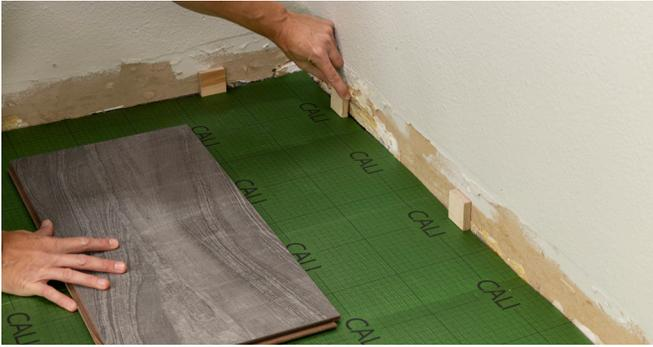
1. Starting from the left, place the first plank with the tongue side facing the wall. Throughout the entire installation process, remember to check that your spacers are maintaining the 1/2" expansion space along room perimeter or next to any fixed objects.
