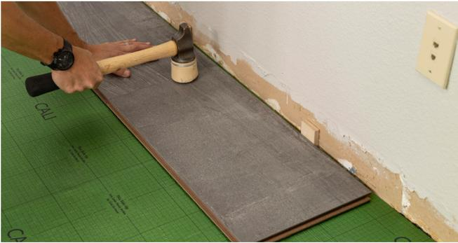
3. Ensure that the planks remain aligned and the joints stay securely closed throughout the installation process. Continue in this manner until reaching the final board in the first row.
