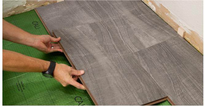
2. Install second plank by angling long side of the plank and gently sliding until the butt end seams are in contact, and then gently tapping all seams into place. After installation is complete remove all 1/2" spacers and insert 3/8" compressible PE foam backer rod. Seal expansion space with 100% flexible silicon sealant. DO NOT use acrylic-based sealant.
