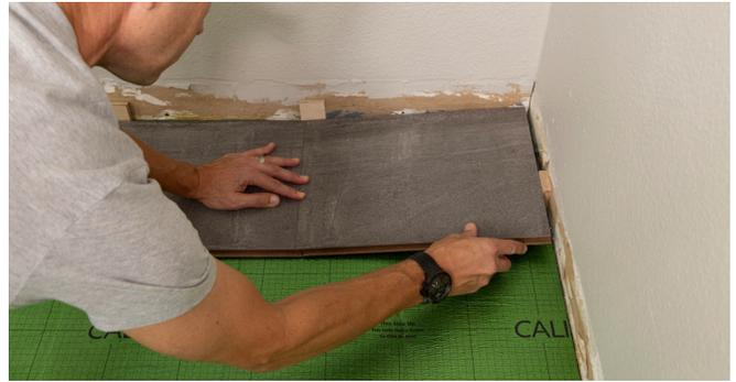
4. When you reach the wall, cut the tile no less than 6" to fit while maintaining the 1/2" expansion gap.
