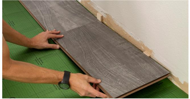
2. Install the second piece by aligning the butt end with the end of the first piece at an angle. Gently push the second piece down until the tongue and groove lock together to secure the end joint. The planks should lay flat.
