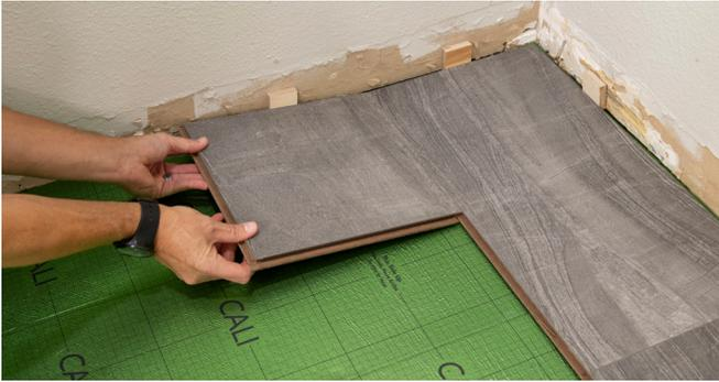
1. Start new rows with pieces trimmed from previous rows that are at least 12" in length and ensure a minimum end joint offset of at least 1/3 the length of the plank. At a slight angle, insert tongue into the groove of the plank from the previous row until the laminate edges meet. Angle down until the joints lock.
