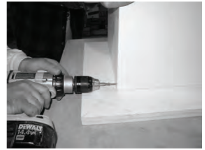
15) Screw or nail final panel to secure in place.
