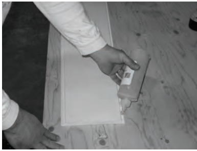
13) Apply adhesive to final panel.
