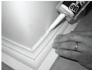
20) Caulk using latex caulking compound to fill any gaps and nail or screw holes.
