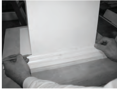
17) Use column shaft to check length of base trim molding. If trim is too long, mark cut lines for miters.
