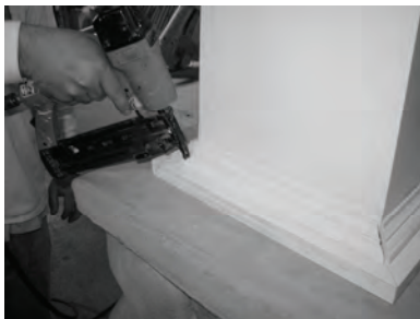
19) Apply adhesive to base trim moldings and pin-nail into place.
