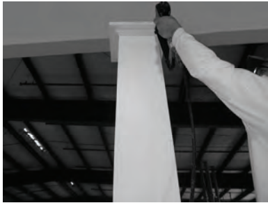
16) Apply glue to final ¼ cap piece and biscuits and slide into place. Pin nail cap moldings to top of column.*
