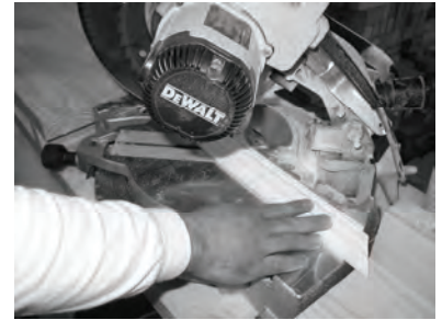
18) If base trim moldings are too long, use miter saw to cut base trim pieces to fit around bottom of column.
