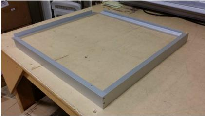
4) Repeat at  $2^{nd}$  corner then attach to ceiling before installing LED panel
