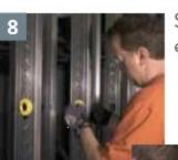
Snap in grommets for electric and plumbing.
