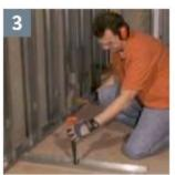
Attach floor runner using concrete anchors.
