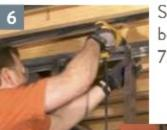
Screw studs to top and bottom runners using 7/16" pan screws.
