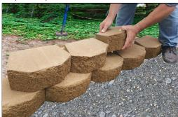
Begin placing the second course of block at straight wall areas being sure to center each unit over the joints of the blocks below in a "running bond" or 1 over 2 pattern. Lips on rear of block should be facing down. Fill backfill area behind wall (see cross section) with clean, crushed stone/gravel for proper drainage. Do not use pea gravel. Proceed to the next course of block, backfilling and compacting as you progress. Repeat until final height is reached to complete wall.
