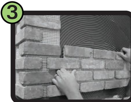
Apply brickweb sheets by over-lapping exposed webbing. Firmly press brickweb into adhesive.
