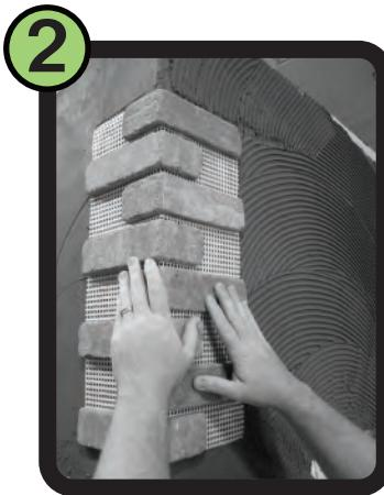
Begin layout process by applying brickweb corners. Firmly press brickweb into adhesive.
