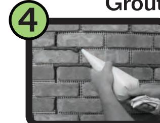
Apply grout using grout bag.
