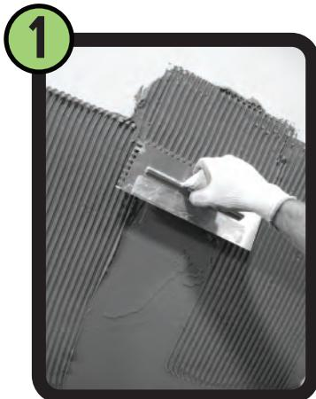
Apply adhesive to substrate using  $\frac{1}{4}$ " x  $\frac{1}{4}$ " notch trowel.
