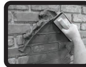
Apply grout using tile float.
