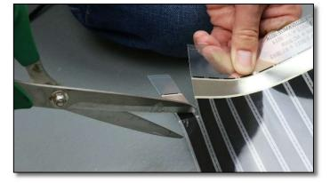
Cut through the last black heating element bar to remove the end of the silver bus bar, creating a notch. Do not over-cut into the next black bar. Repeat on both sides.
