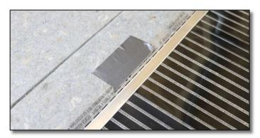
Lay the mats out according to your design plan and tape in place with a high quality duct tape on the sides. This step is just to hold the mats in place while you continue working in the area. You don't need to tape on the ends. There is no "top" or "bottom" to the mats.
