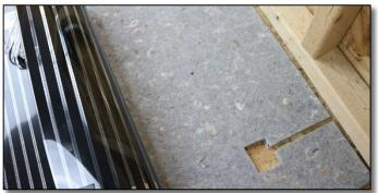
If you used an underlayment, cut a channel for the power supply lead wires and connections out of the underlayment. If there is a vapor barrier below your underlayment, be careful not to cut the vapor barrier.
