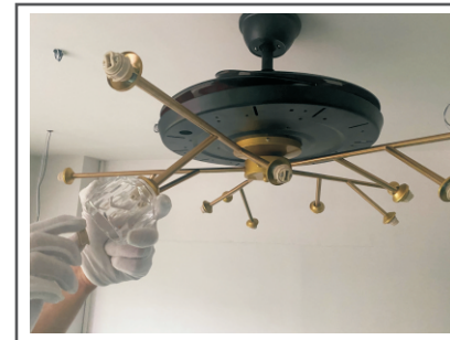
Step 6. Install crystal lampshades.
