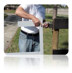
Drop the bearing into the barrel and place the smooth end of the J Bolt into the hinge barrel. Hold the gate frame the height off the ground you would like your gate to hang and hold the hinge plate against the post and mark its position.
