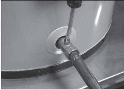
Figure 10 - Draining the old water heater.
