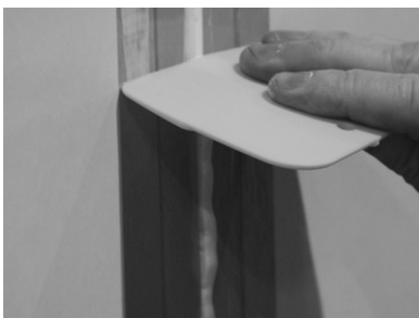
FIGURE 18: REMOVING EXCESS SEALANT
