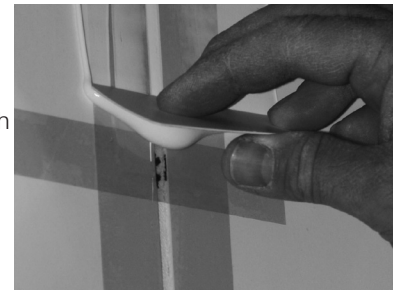
FIGURE 17: APPLYING THE PAINTER TAPE HORIZONTAL IN 3' SECTIONS
