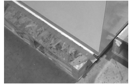
FIGURE 22: HORIZONTAL SEAM FILLED COMPLETELY WITH SEALANT
