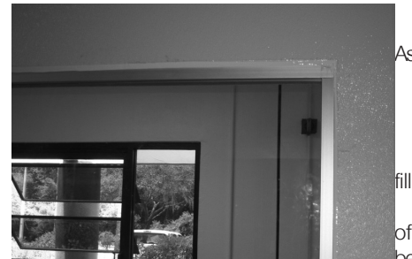
FIGURE 24: TYPICAL WINDOW SEAM APPLICATION
