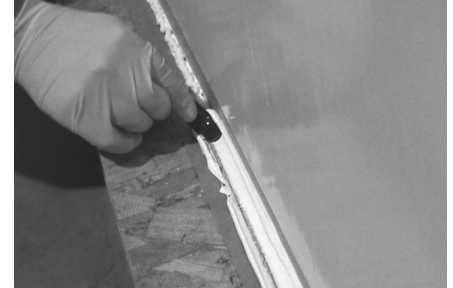
FIGURE 23: HORIZONTAL FINISH WITH ROUNDED CORNER
