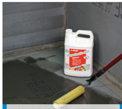
With a roller or brush, apply the primer.
