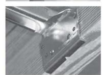
Two barbs on each side of brace will hold brace into position. Secure brace into wood with four, # 12-14 X 1" long lag screws.
