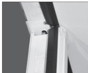
FIGURE 14: Correct sagging until the flush bolt slides freely into the pre-drilled hole (not typical of most units) in the head/threshold.
