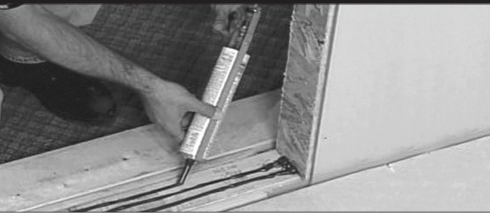
FIGURE 2: Caulk is applied in three parallel lines running the width of the sill.
