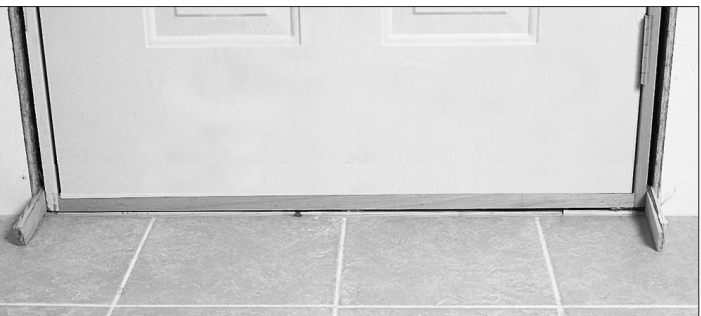
FIGURE 11: Proper position of shims at the bottom of the door (Points A).
