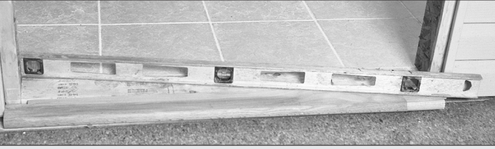
FIGURE 1: A clean, level, solid sub-floor area is essential to successful installation.
