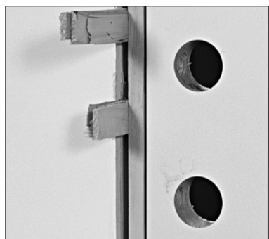
FIGURE 12: Shims are placed above and below the dead bolt hole (points G in Figure 10).
