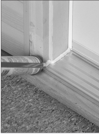
FIGURES 24 and 25: Caulk the sill crown and the front of the sill.
