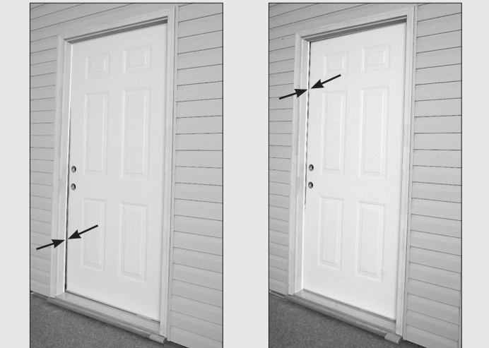
Figures 8 and 9: The weather-stripping on these doors is not evenly compressed.
