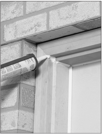
FIGURES 26 and 27: Caulk the jambs and the exterior trim.
