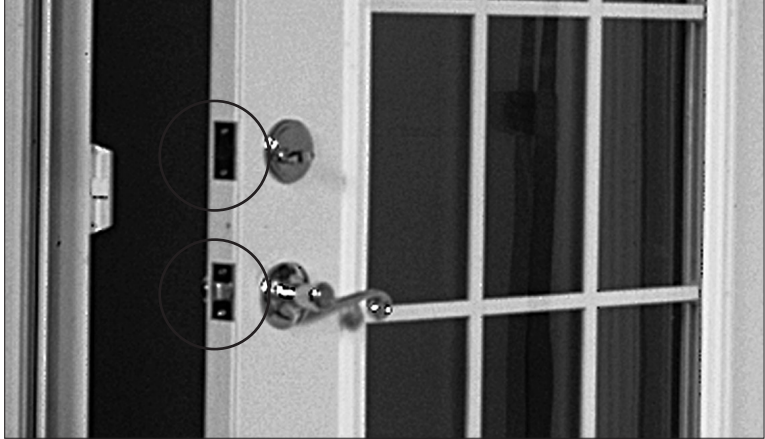
FIGURE 29: The latch and dead bolt are installed per the hardware manufacturer installation detail.
