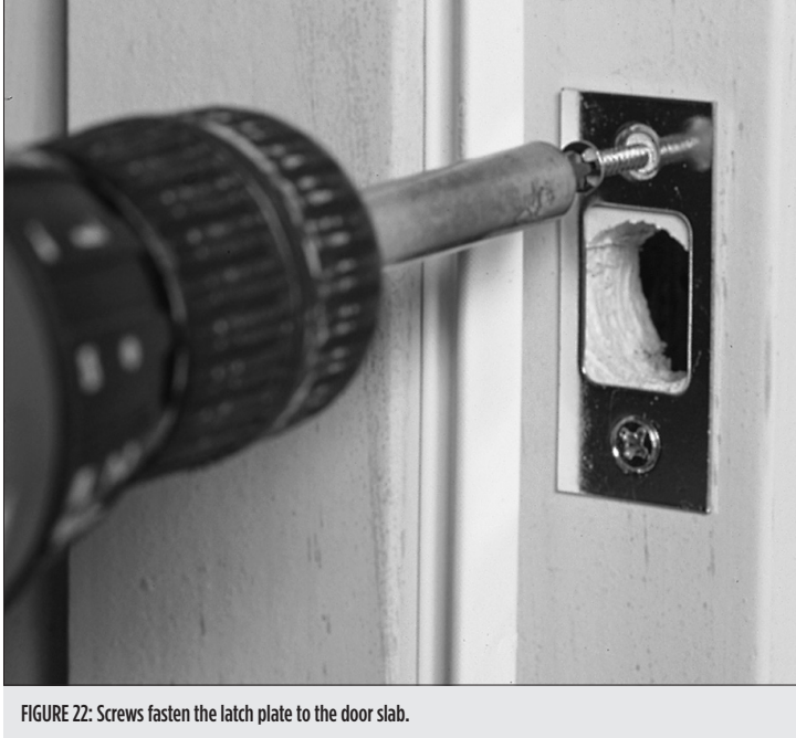
FIGURE 22: Screws fasten the latch plate to the door slab.
