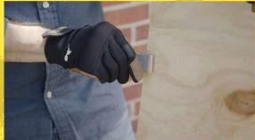
Slide PLYLOX<sup>™</sup> window clips on to opposing vertical edges of the plywood cover and make sure it fits tightly.
