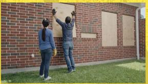
With the teeth towards you, against the brick, push the plywood sheet into the window casing.
