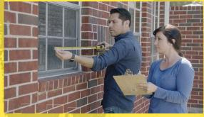
Measure the height and width of a window. Subtract 1/4" from each measurement leaving 1/8" clearance.
