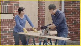
Cut your plywood 1/4" smaller that the window opening which allows 1/8" clearance all around.
