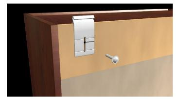
e. With the cabinet mounting bracket alignment leg resting **flat against the cabinet top**, tighten the screw so that the T-nut barbs engage the face of the cabinet interior rear surface. Repeat for the other cabinets. If you plan to use the decorative plastic T-nut covers, you can install them at this point.
