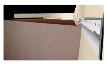
c. Make sure that the cabinet brackets have engaged the wall rail before releasing the cabinet.
