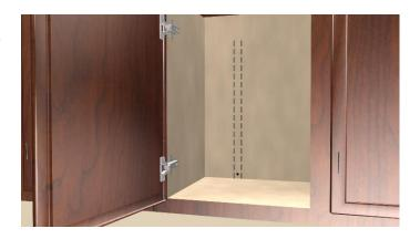
c. Again, using the provided horseshoe style shims for spacing, install  $10 \times 2 \frac{1}{2}$ " washer head screws through the cabinets' lower sections. The combed design allows them to slide up along and hold onto the bottom screws while adjustments are made.
