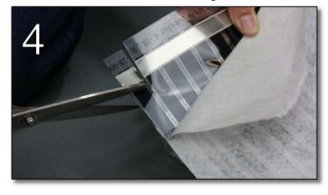
Cut through the last black heating element bar to remove the end of the silver bus bar, creating a notch. Do not over-cut into the next black bar. Repeat on both sides.
