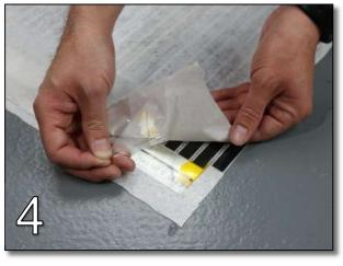
Once the heating element is adhered to the bottom of the flap carefully peel back the upper release liner and press down to seal the edges of the membrane.
