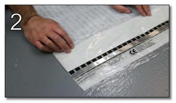
Lay back the white flaps on the long sides of the mats to expose the clear film with metal conductor bars and black heating elements.
