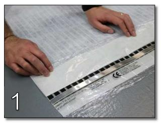
Fold back and crease the top white "flap" on the side of the heating panel to keep it out of the way while working with the bottom flap.
