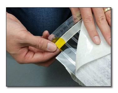
Use the included Kapton discs to insulate the cut ends of the silver bus bars. The silver bus bars run parallel down the length of each side of the mat and are the electricity conducting component of the mat.
