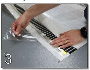
Peel the release liner on the bottom flap to expose the adhesive. Lay the heating elements down on the bottom flap and press with your hands, smoothing out all air bubbles.
