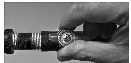
Figure 58 - Gas valve in “on” position.
