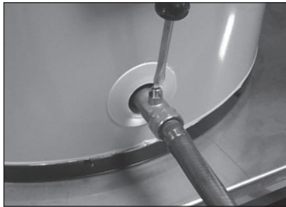
Figure 10 - Draining the old water heater.
