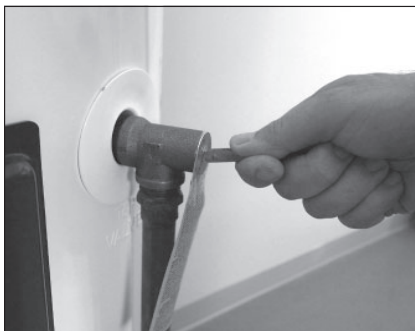
Figure 41 - T&P Relief Valve
