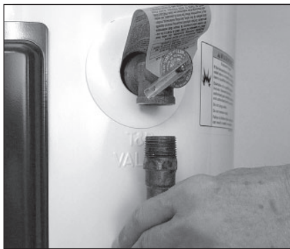
Figure 11 - Removing the T&P Relief Valve discharge pipe.
