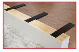
3. Once the "pocket" is made in the knee/pony wall, simply insert the bracket then screw the bracket into place making sure your screws are flush with the brackets.
