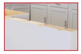
1. Mark 3"-6" from the outer edge of the knee/pony wall for your first pocket to be cut. Then set marks for the remaining brackets every 16"-20" apart for the best counter top protection.
