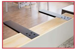
4. Using a level, make sure your brackets are level; use shims where necessary until the brackets are completely level.
