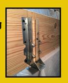
Step 2: Use a nail gun to secure the joist hanger to the ledger board.
