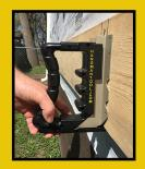
Step 3: Pull off the Hang Em Fast, leaving just the joist hanger.
