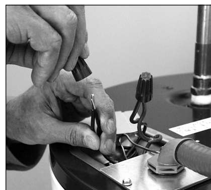
Figure 19 - Connecting the electrical wires.
