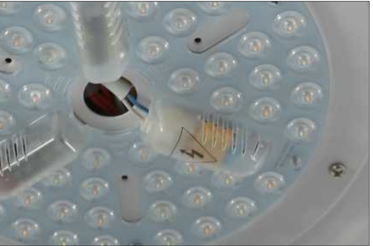
Step 19 Connect the light kit power cord to the light kit receiver.
