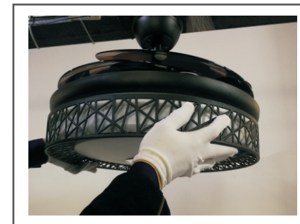
Step 5. Install the lampshade counterclockwise on the chassis of the main fan lamp.
