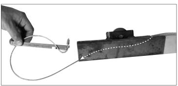
8a. Reload and insert the cable installation tool into the BOTTOM end of the "B" section as shown.
