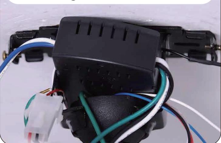
35. Lift the canopy into place and wrap keyhole slots around the screws
