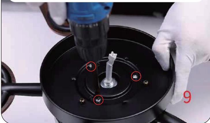
10. Remove the three light kit screws on light plate
