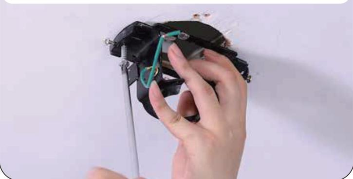
29. Place the downrod ball into the ceiling bracket. Be sure the fixation slot is locked by the bracket. If not, rotate the ball until the fixation slot is locked
