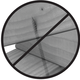
Incorrect installation with SDWC Truss screw protruding out the side of rafter/truss
