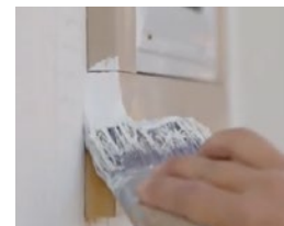
Prime Exposed Raw Edges before Top Coating
