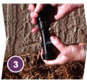
3) Next, attach the 150 mesh-screen Filter (helps keep drippers clog-free) 4) and the 1/2-in Poly Faucet Fitting.
