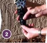
1) Begin by attaching the Backflow Prevention Valve to any outdoor faucet. 2) Then attach the 25 PSI Pressure Regulator (reduces water pressure to optimal levels).
