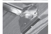
Two barbs on each side of brace will hold brace into position. Secure brace into wood with four, # 12-14 X 1" long lag screws.
