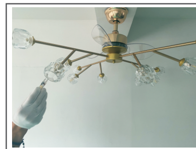
Step 8. Install the G9 light source
