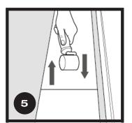
Use a resilient flooring hand roller to squeeze out any remaining adhesive in tight spaces.
