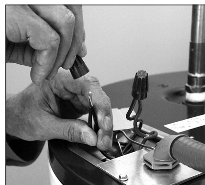
Figure 19 - Connecting the electrical wires.
