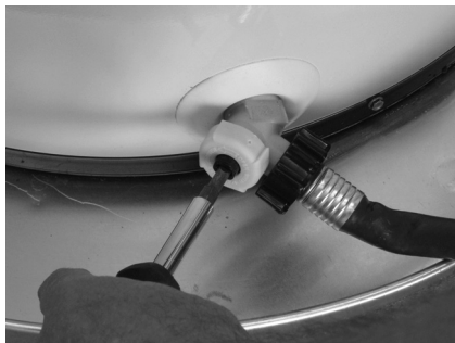
Figure 10 - Draining the old water heater.
