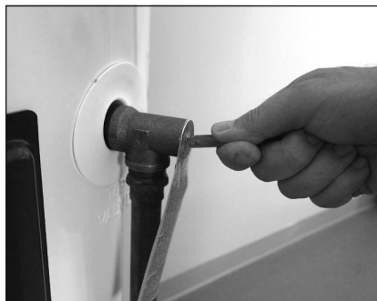
Figure 38 - T&P Relief Valve
