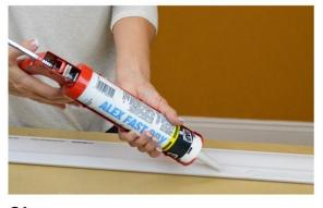
**Glue**Glue with a water-based painter's caulk.
