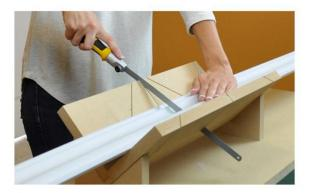
**Cut**Material is easy to cut with a simple saw.
